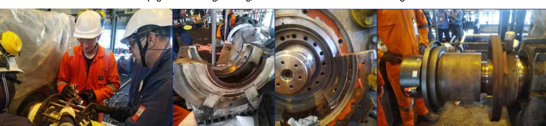
Generator rotor testing, extraction, re-installation, stator repair, cryogenic cleaning, testing, re-instatement and commissioning
